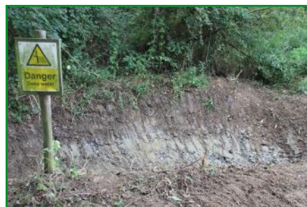
A newly cleared silt trap, Beggar Boys Wetland, September 2018
